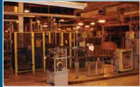
(1 OF 3) AUTOMATION ENGINEERING NO LOAD TEST STATIONS
