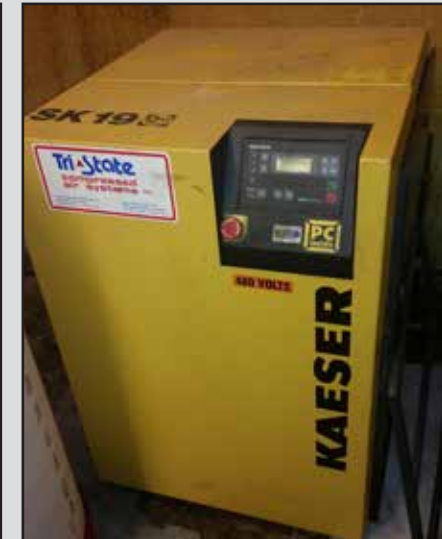
KAESER SK19 AIR COMPRESSOR
