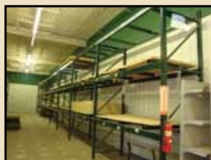
OVER 50 SECTIONS OF PALLET RACKING
