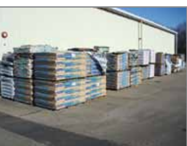
HUGE QTY. OF ROOFING MATERIALS
