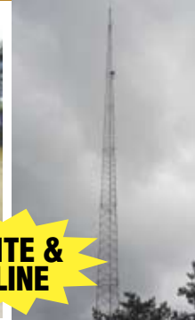
COMPLETE 180' RELAY TOWER SYSTEM
