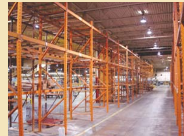
(Over 500) Sections Of Various Pallet Racking
