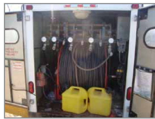
INSIDE OF THAWZALL SYSTEM
