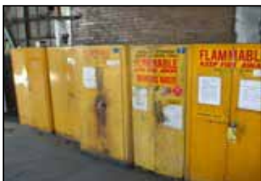
FLAMMABLE STORAGE CABINETS
