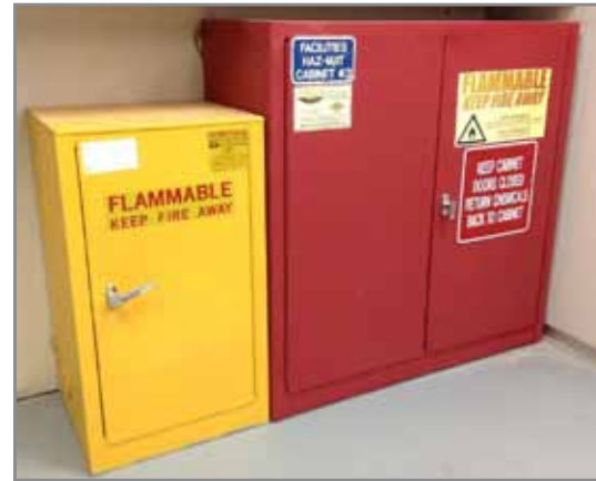
(10) FLAMMABLE LIQUID STORAGE CABINETS
