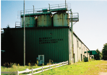
Front of the facility
