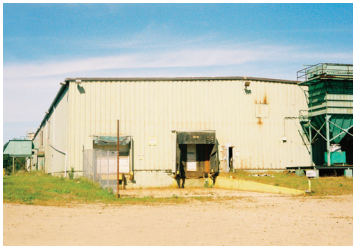
Rear of the facility
